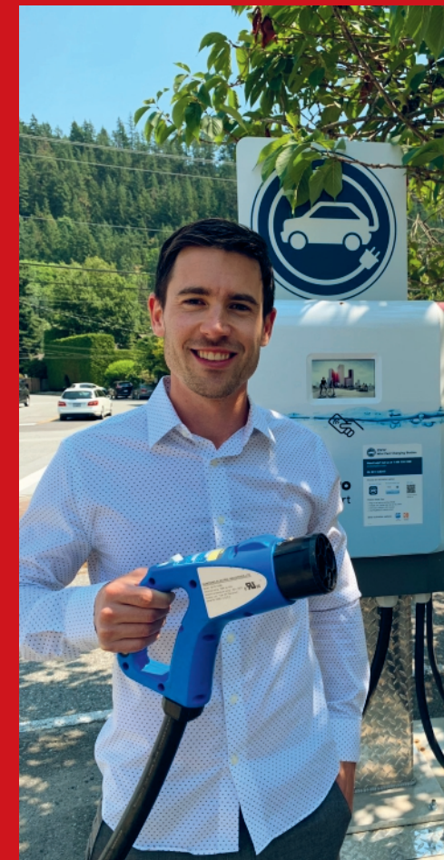
EV charging station in Horseshoe Bay
