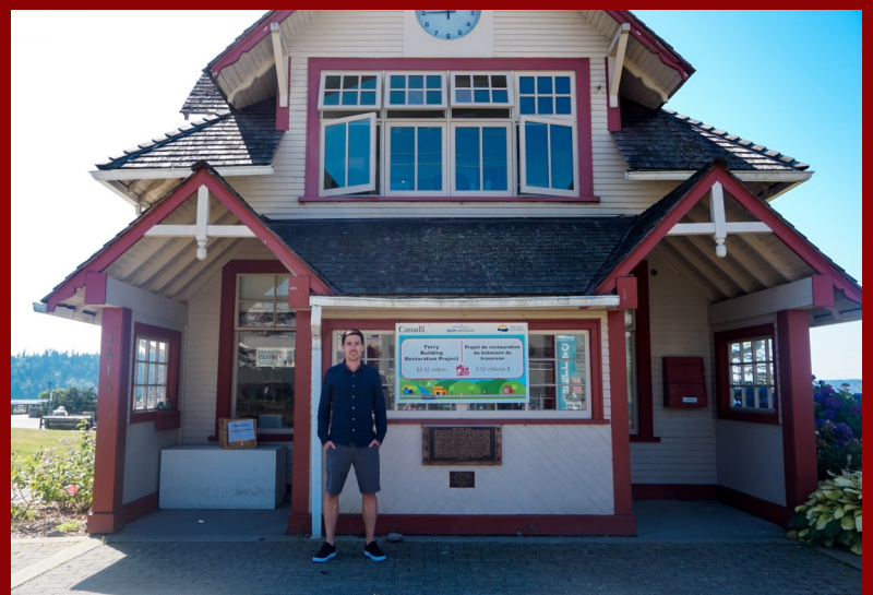
Photo: West Vancouver Ferry Building Restoration Project.
